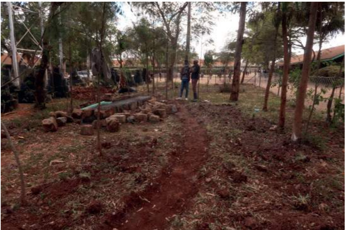
Pathway and bench under construction
